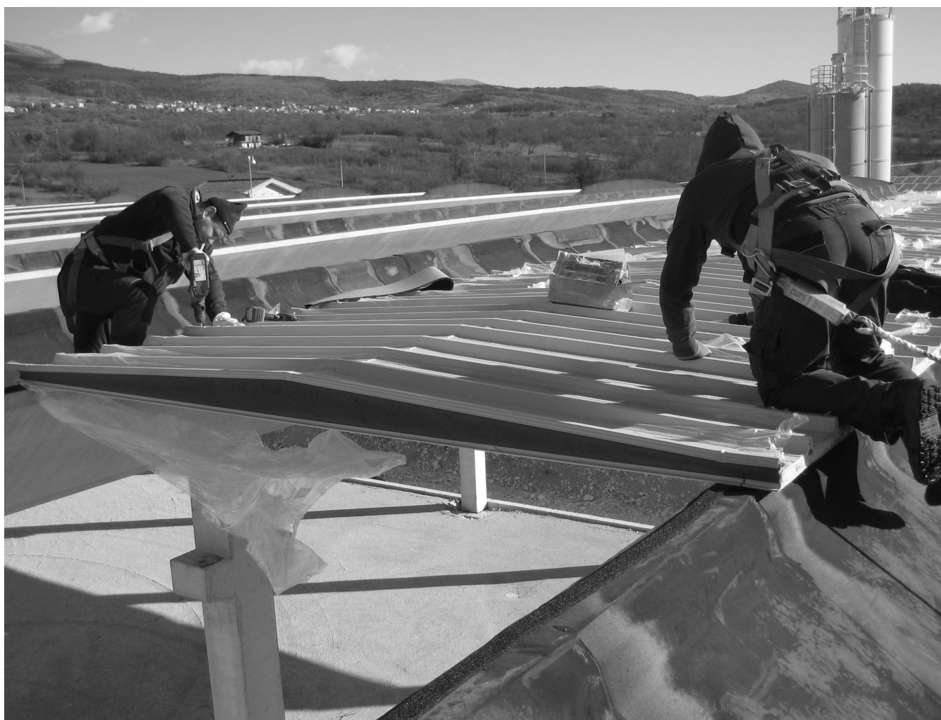
Picture n° 11: laying of the TECHTUM panel on reinforced concrete wing beams
